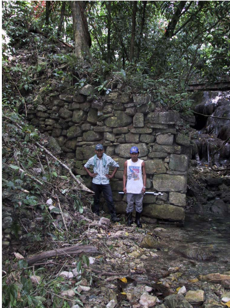
Figure 2.11 Photo of the Group C Bridge's eastern pillar.
