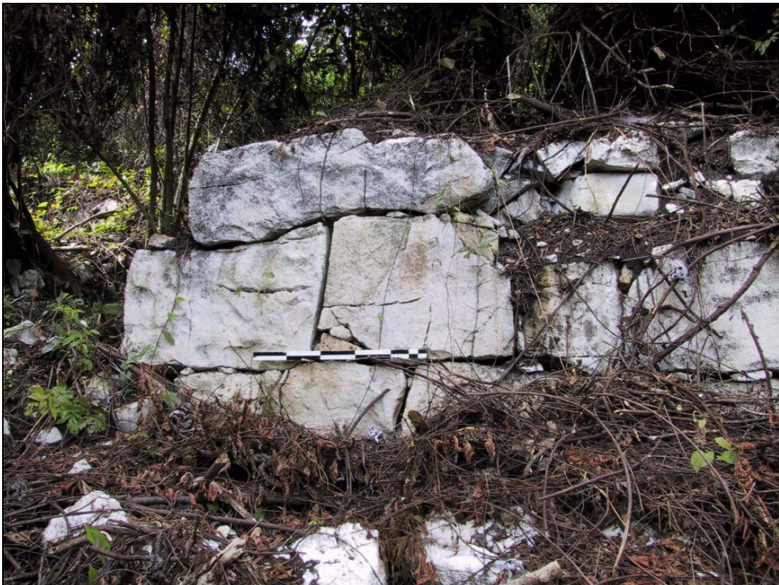
Figure 2.6 Photo of Structure Y27's northeast corner.
