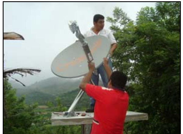
Satellite dish being installed at the Yaxalum Dormitories
